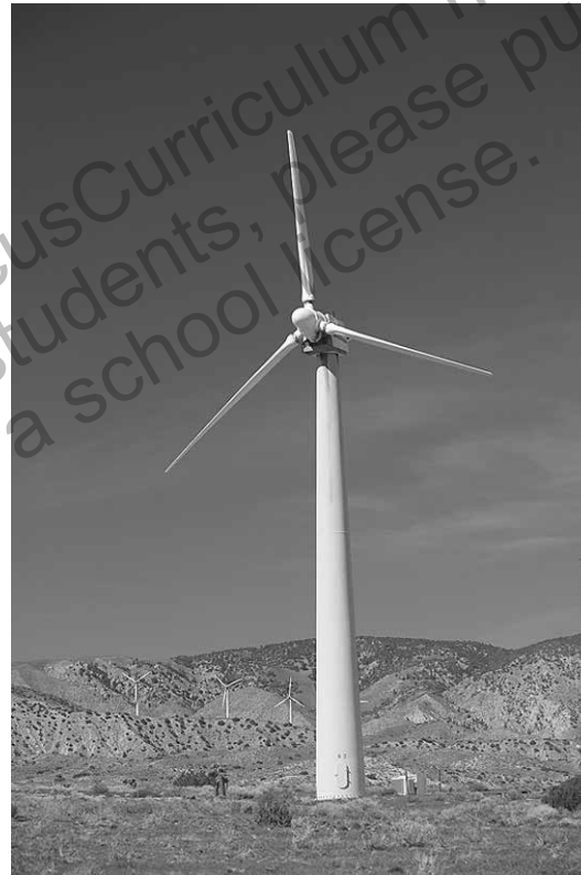
A typical wind turbine has blades, a generator, and a computer system to control the blades.
